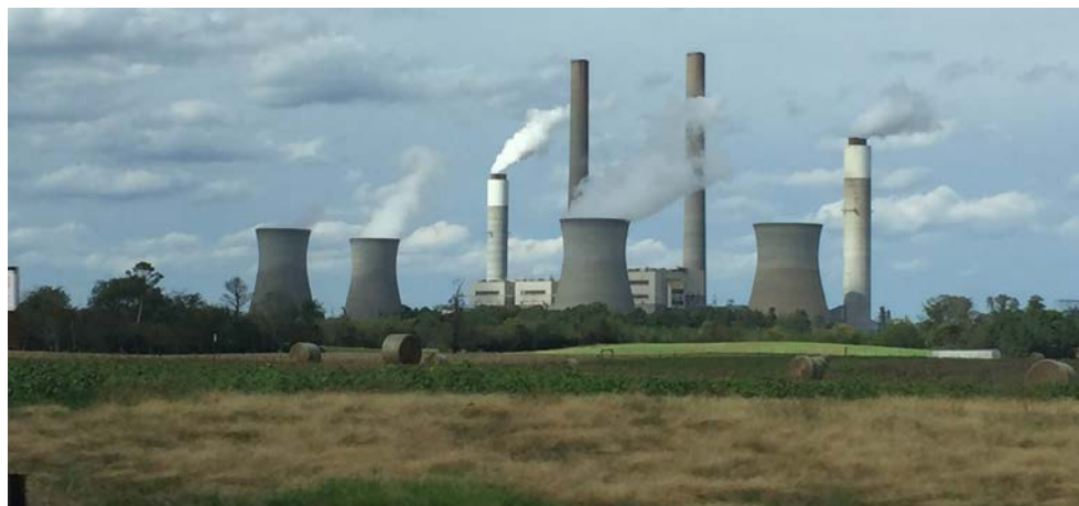
Figure 10: Georgia Power's Plant Bowen - site of the WRC
