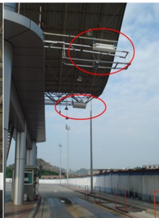
Figure 4 checking bridge of port
