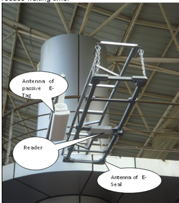
Figure 3 Antenna of E-Tag and E-Seal and reader
