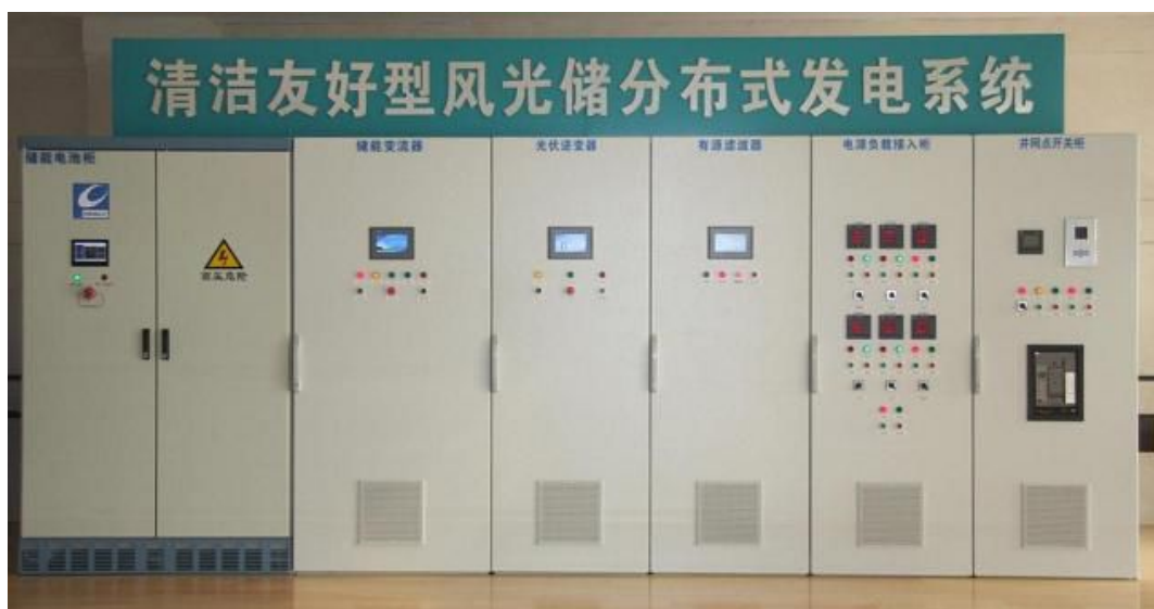
Fig.5. 10 Clean-friendly Wind-photovoltaic-energy-storage Distributed Power Generation System
