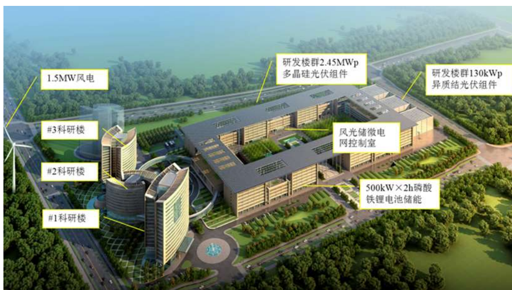
Figure 1:Guodian New Energy Technology Research Institute's wind-solar storage system study distribution schema
