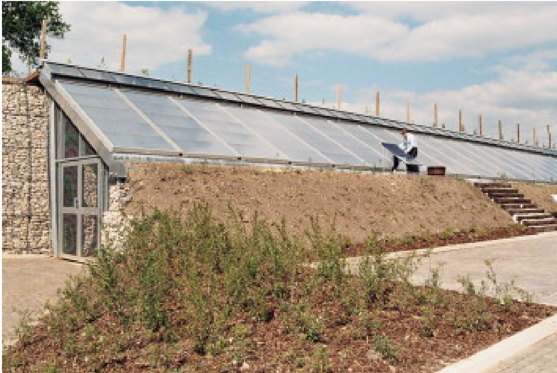
Fig. 2.1. PVT façade at RES UK in Kings Langley (UK). Photograph © Henk Kaan.
