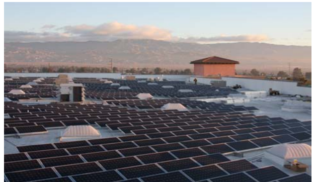
Solar PV on a Wal-Mart in Palm Desert, CA. Photo courtesy of BP Solar.
