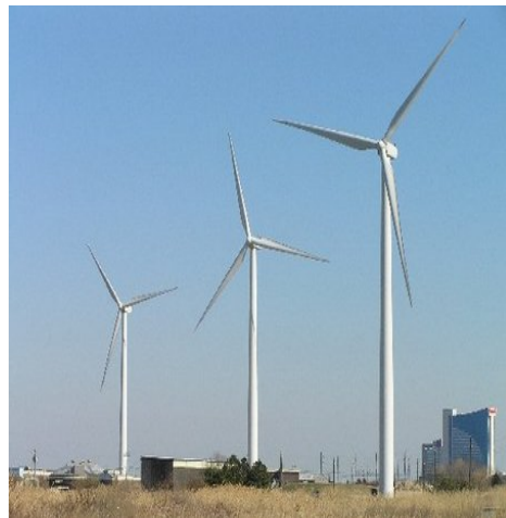
Figure 5-2: 7.5 MW Urban Windfarm, Atlantic City, NJ (USA).
