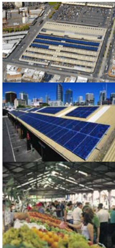
Photos illustrating the solar installation at the Queen Victoria Market. Courtesy of New York City Climate Summit
