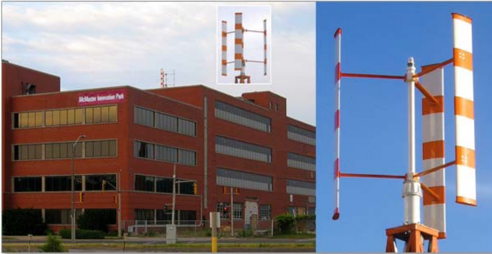
Figure 2-7: V3.5 Installation at McMaster University, Innovation Centre, Hamilton, Ontario, Canada
