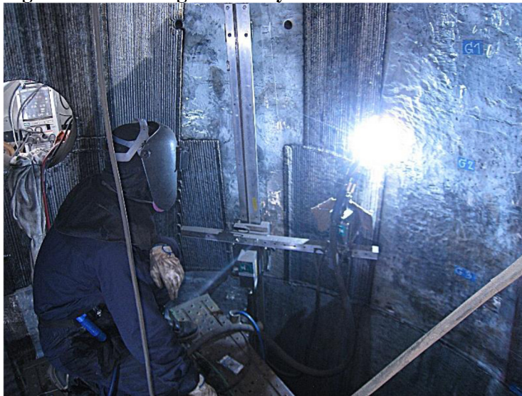
Figure 3.1. Cladding under way
