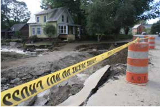
Photo: Homes and Vermont Route 107 (VT) 107 in Bethel, VT near the White River were damaged by quickly rising water during the Hurricane Irene flood event. photo credit: Ann Froschauer/USFWS Source: courtesy of Wikimedia Commons
