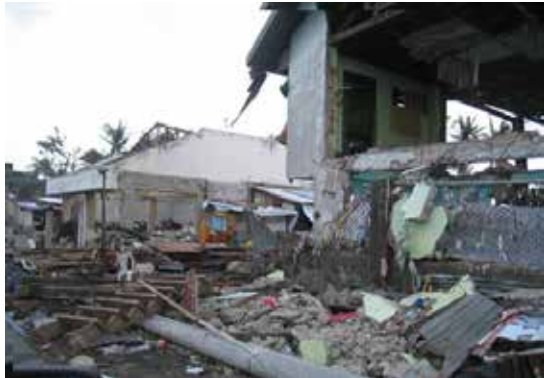
Photo 1: Devastation on the structures
