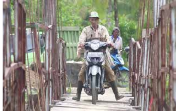
Photo 5. Bike and pedestrian bridge in the Nemnemleu Monga-Mentawai District of South Sipora
