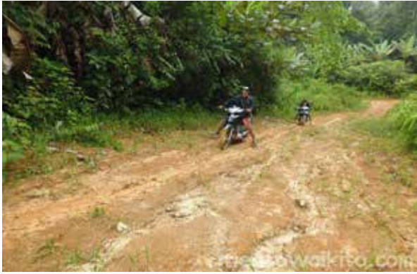
Photo 4. The Large bridges were damaged in the South Siberut village of sub-district in 2014
