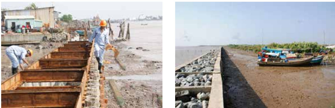
Photo 2. Low cost and “soft” technology applied for sea dike embankment (Source: PMUARDW, 2017)
