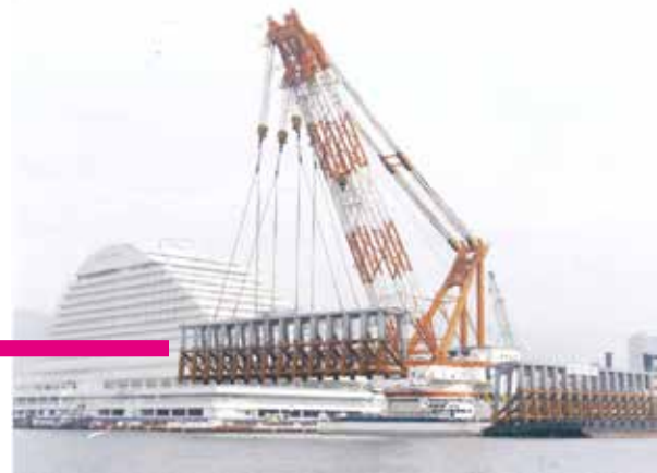
Photo and figure: application of the “steel jacket method”
