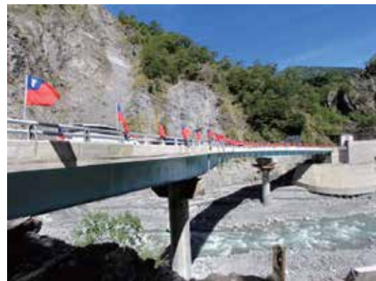
Photo 1-2 Reconstruction of the new Lidao bridge
