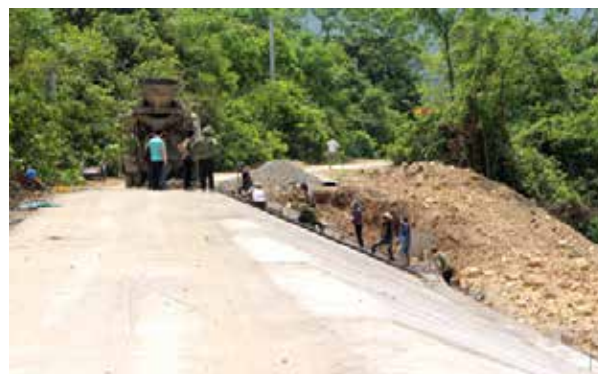
Photo 4. The road under construction
