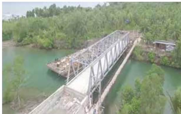
Photo 3. The new bridge to Monga village, next to the old bridge
