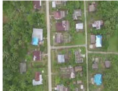
Photo 2. Aerial View of Trans-Mentawai road splitting the village
