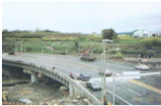
Photo 2. Reconstructed Shihwei Bridge
