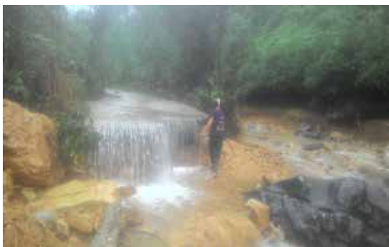
Photo 1. Road damaged by the historic flood
