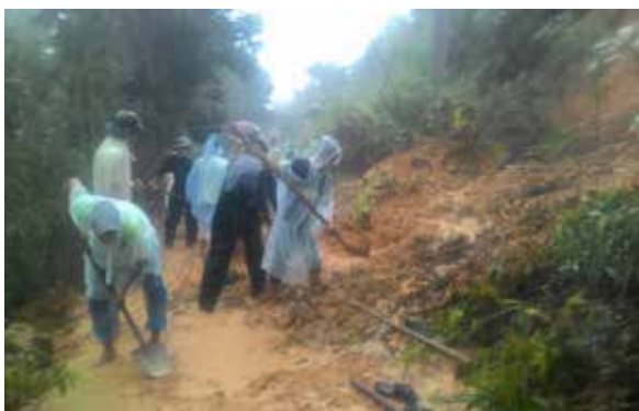
Photo 3. Urgent and rapid repair of the road in the disaster
