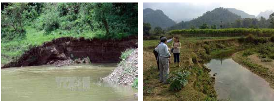
Photo 4. Land erosion and sliding at the banks of Thanh Mai stream near Ban Phat village, Bac Kan province Source: MARD-PMU, 2016
