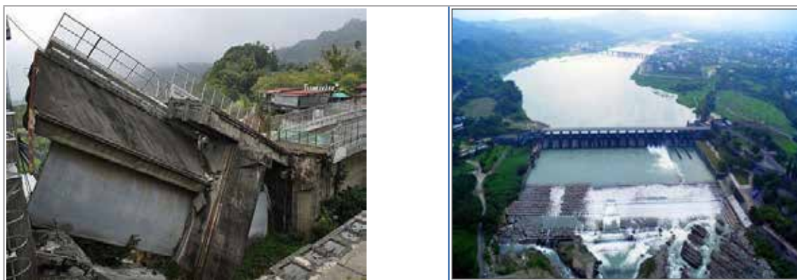
Photo 1. Shihgang dam: (a) after the earthquake and (b) after reconstruction
