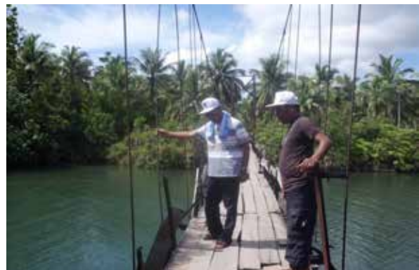
Photo 7. Old Monga Bridge, made of wood with a width of 2 meters
