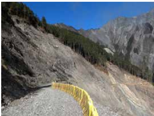
Photo 1-1 The Lidao bridge collapse
