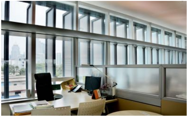
Figure 2 Lightshelves at perimeter office
