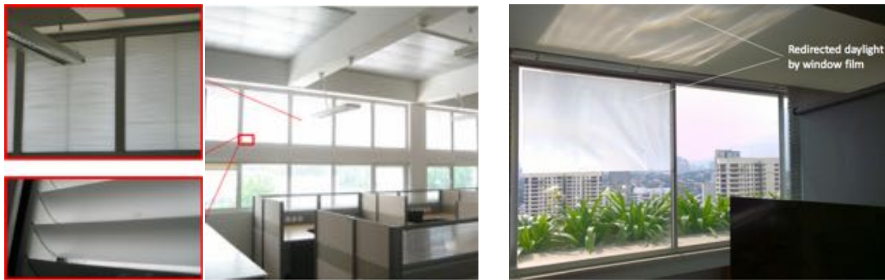
Figure 15 Split-level window and integrated blinds
