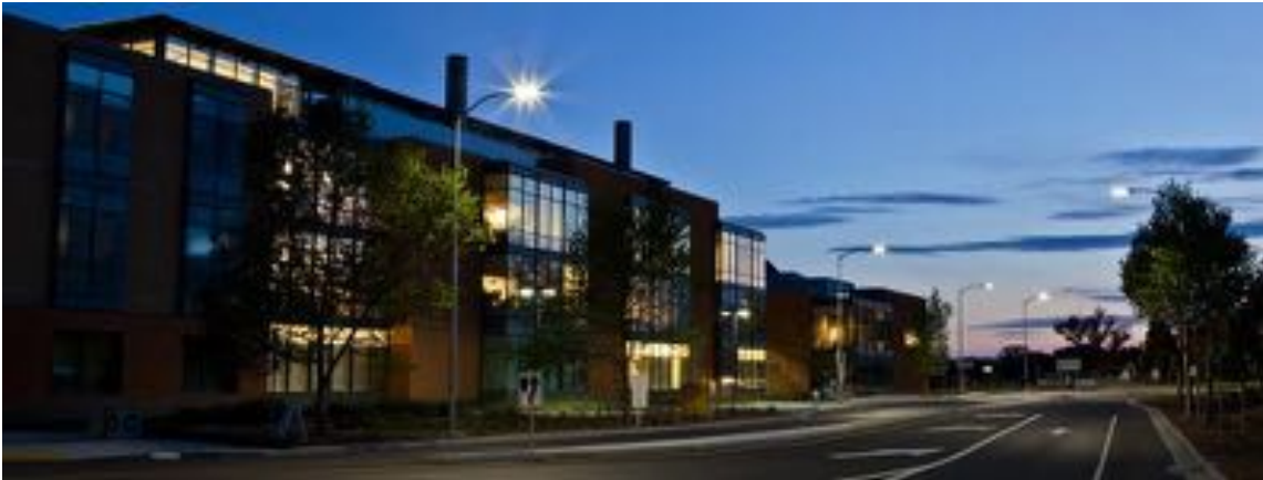
Figure 11 Demonstration of networked street lighting controls at City of Davis (Photo Credit: California Lighting Technology Center)
