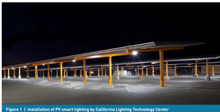
Figure 1 | Installation of PV smart lighting by California Lighting Technology Center
