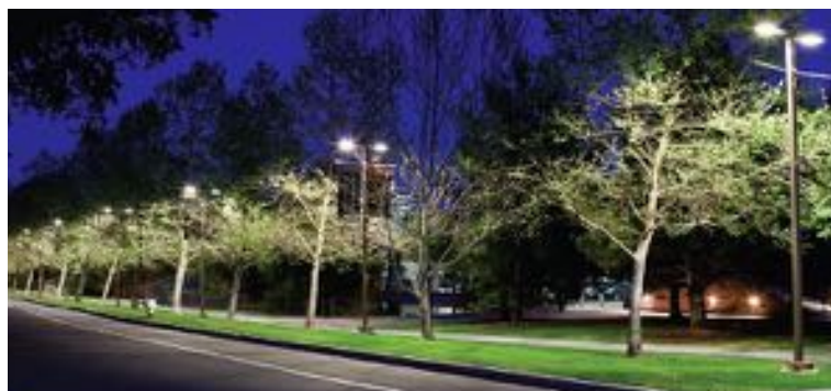
Figure 1 | Installation of adaptive lighting by California Lighting Technology Center
