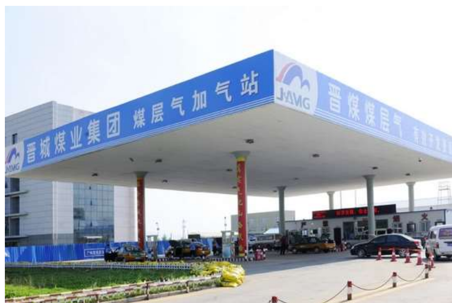
Fig.2-15 CBM filling station in Jincheng
