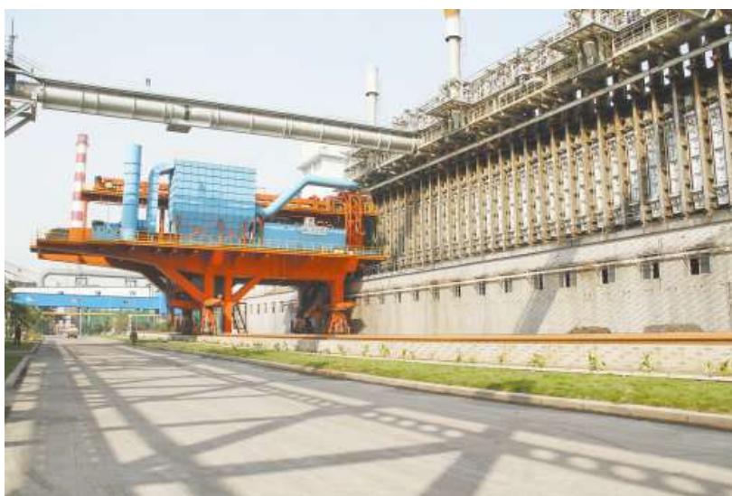
Fig.2-9 7.63m coking furnace of Shoushan Coking and Chemical Company of Pingmei Shenma Group
