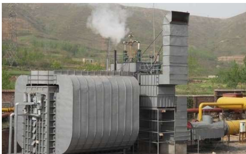
Fig.2-11 VAM oxidation project in No.4 Coal Mine
