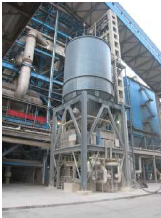
Fig.2-3 Wastewater treatment plant in Yaoqiao Coal Mine
