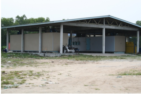
Photo 2.3: Cold storage facilities at the Tok Bali, Kelantan branch of the Fisheries Development Authority (LKIM) fish landing port. These facilities chill fish down to -20 Celsius. The facility is not utilised as most landings go straight to market. Photograph taken August 2008.
