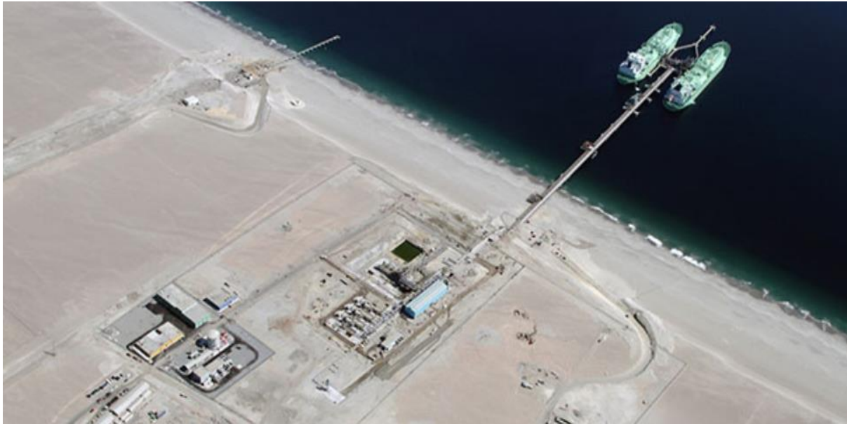
Figure 28: Chile Mejillones LNG terminal with FSU 58
