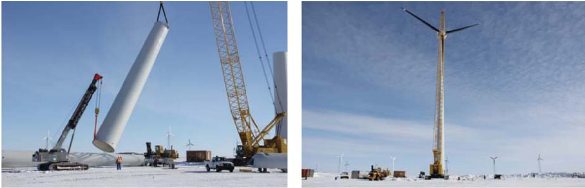
Figure 4. Installation of an EWT 900 wind turbine
