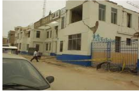
STRUCTURAL COLLAPSE OF HOSPITAL - ESSALUD (SOCIAL SECURITY) PISCO - PERU 2007
