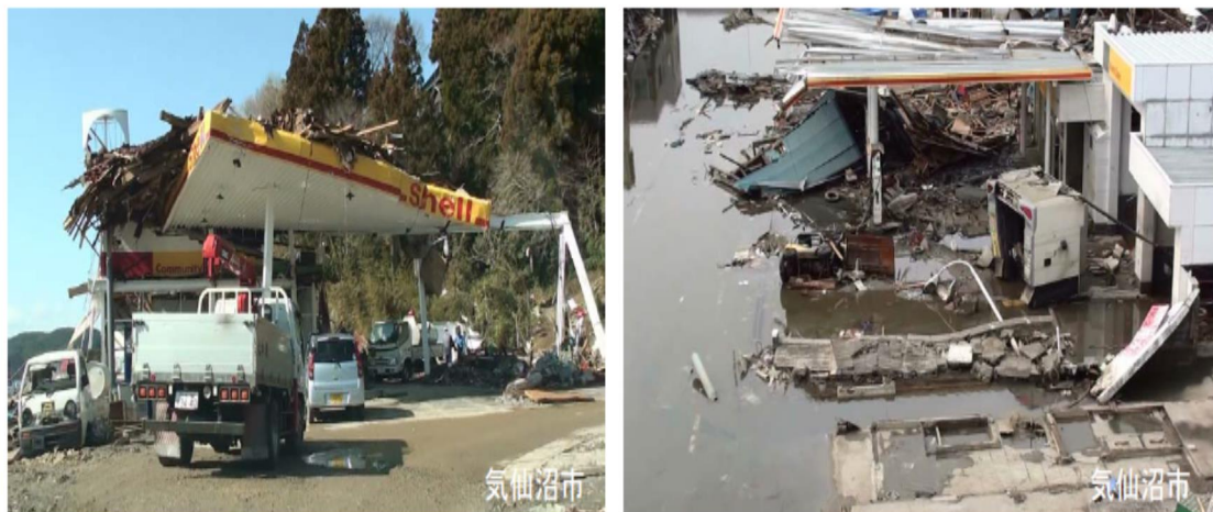
Figure 3 (Damaged service station in Kesenuma City)
