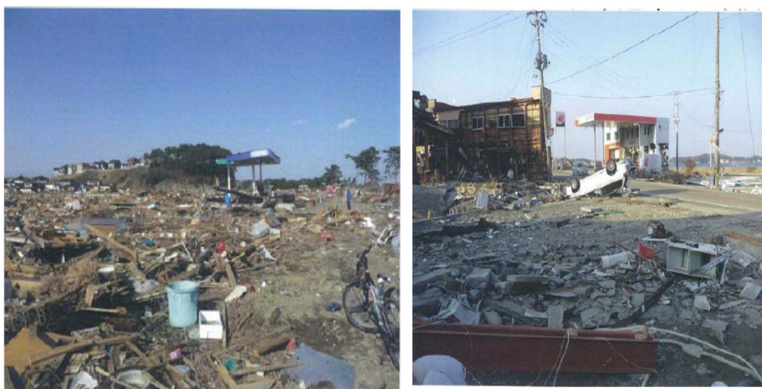
Figure 4 (Damaged service station in Shichirigahama, Sendai City)
