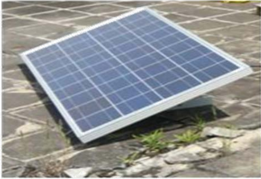
Fig. 4.2 Fixed solar panel system
