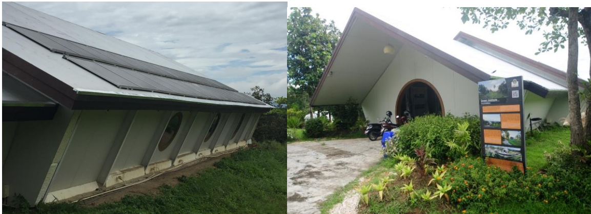
Figure 5. 3 Bird House rooftop PV system
