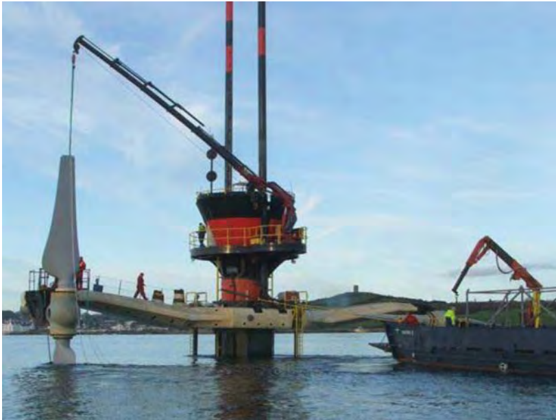
Figure 15. Maintenance of SeaGen: Most maintenance and repair functions can be completed rapidly, using no more than small service vessels. Here: fitting a new rotor blade
