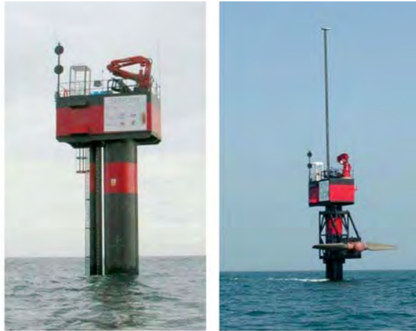
Figure 11. Seaflow, world's first full-size offshore tidal current turbine
