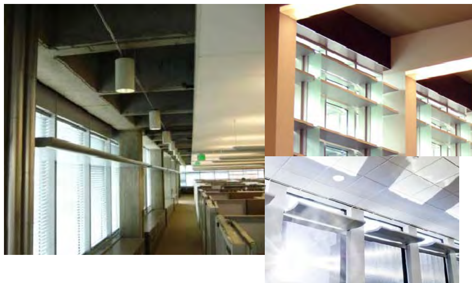
FIGURE 11-22 : Light Shelf for Natural Light Uses
