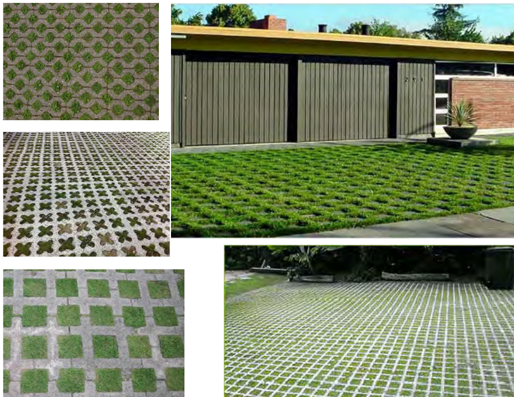
FIGURE 11-25 : Green Paving (Grass Block)
