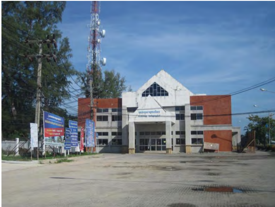
FIGURE 5-10: Kanchanapisek Conference Hall before proposed renovation
