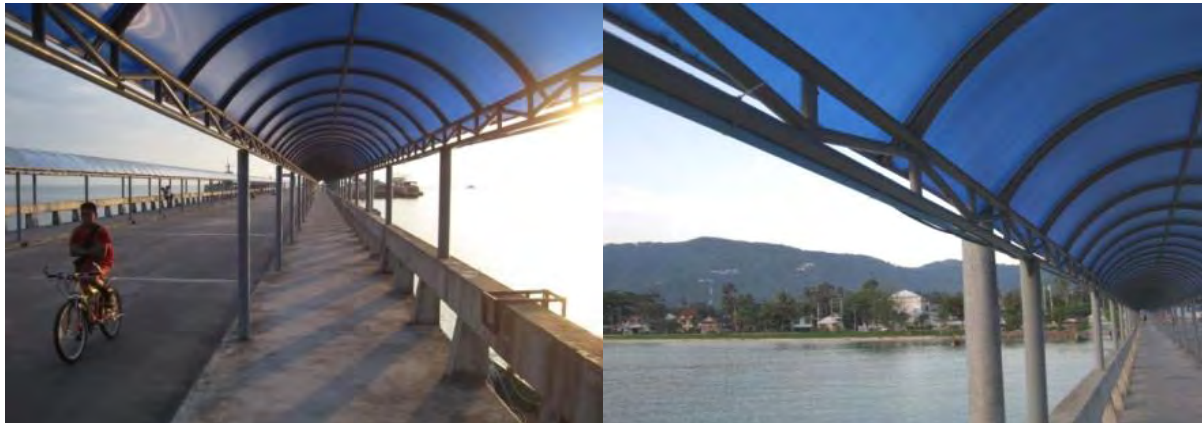
FIGURE 5-22: Covered-ways at municipality's pier 2 (before)
