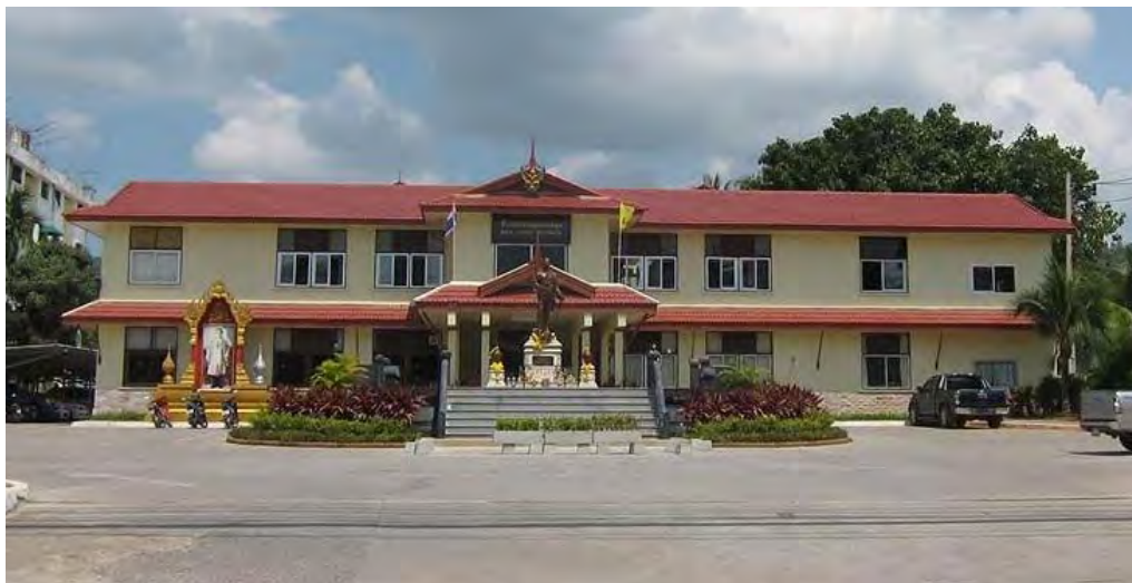
FIGURE 11-18 : SAMUI District Office
