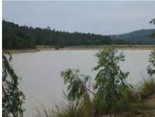
FIGURE 13-2 : Na Muang Reservoir
