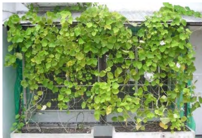
FIGURE 5-25: Wire mesh with climbing plants
