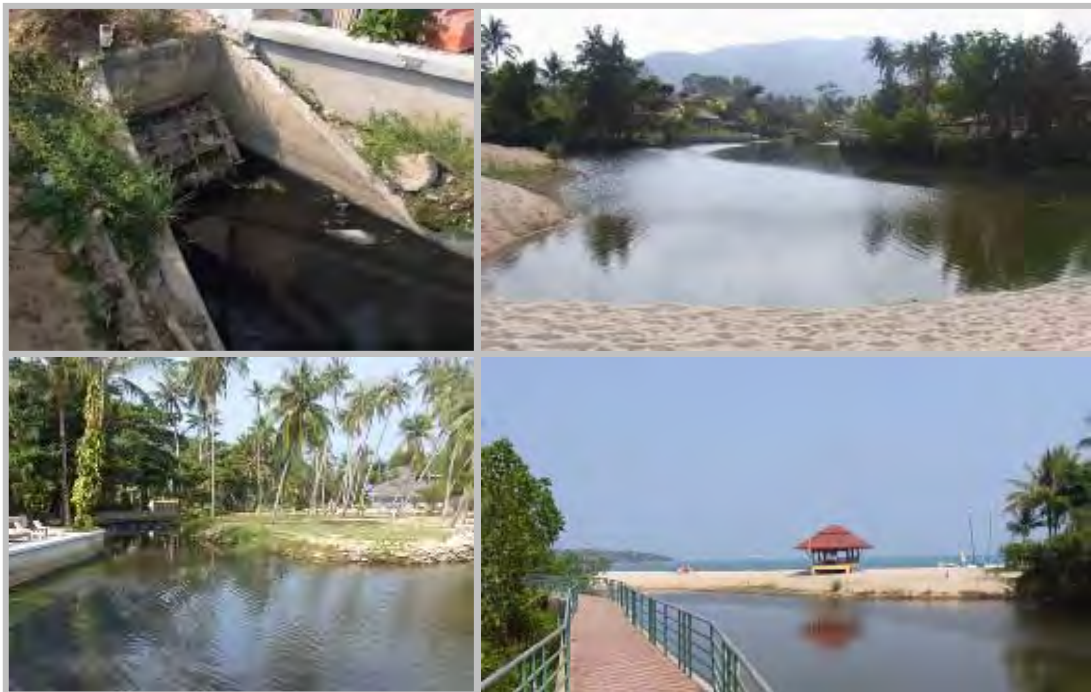
FIGURE 13-11 : Existing wastewater discharge point
