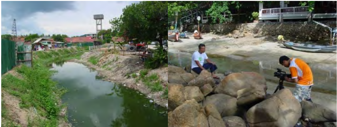
FIGURE 5-6: Conditions of banks of Chaweng canal
