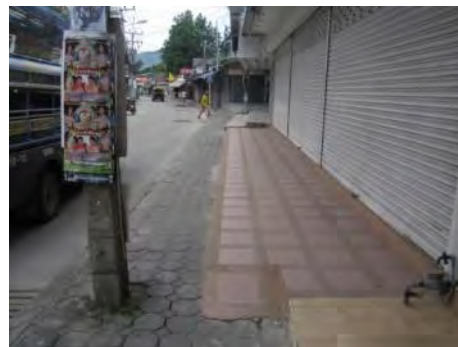
FIGURE 5-91: Uneven, poorly maintained and inconsistent walkways on Chaweng 1 Road
