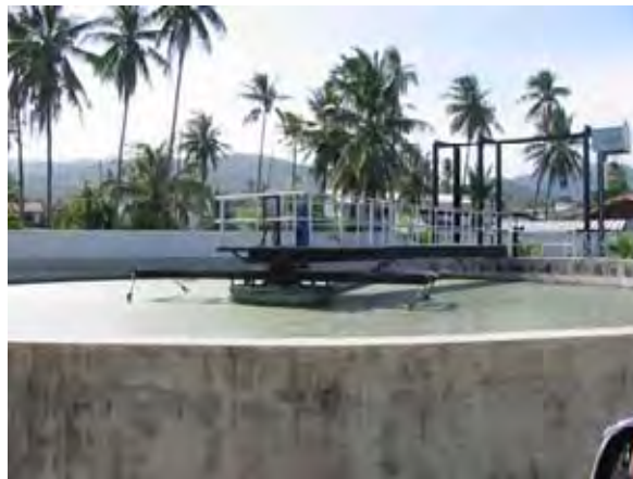
FIGURE 13-22 : Nathon Wastewater treatment plant
