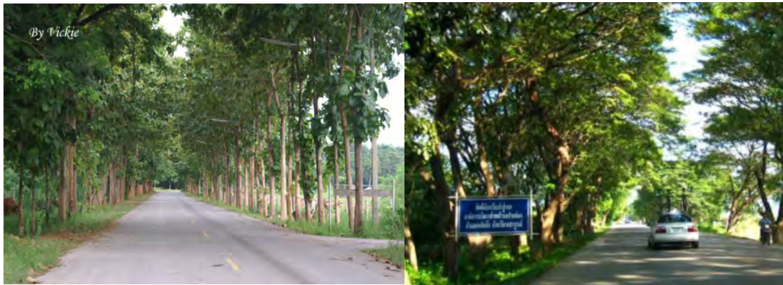
FIGURE 5-31 : Example of greenery state highway
