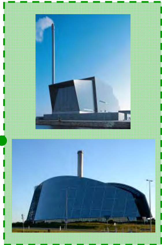
The New incinerator power plant
