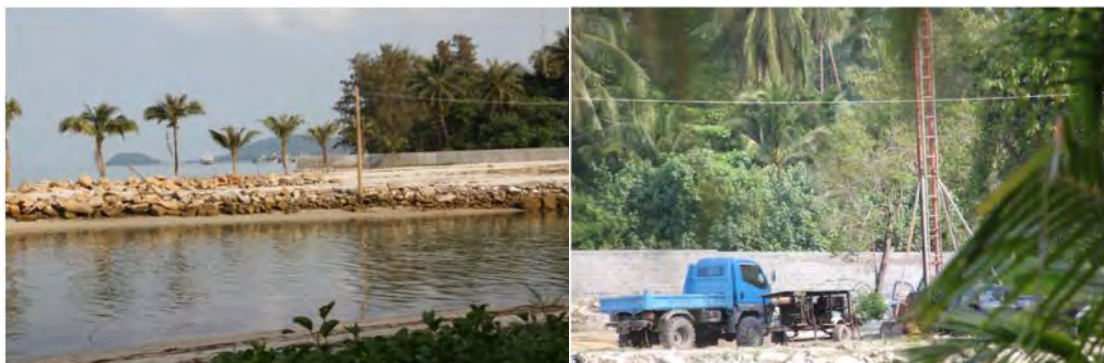
FIGURE 5-5: Construction of leisure place at Lipa Yai canal's estuary
