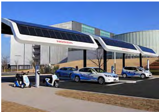
FIGURE 6-17 : Example of charging station ( Saitama City, Japan)
