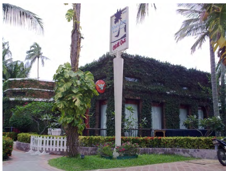
FIGURE 5-9: Green walled building example at Buddy Oriental SAMUI Beach Resort
