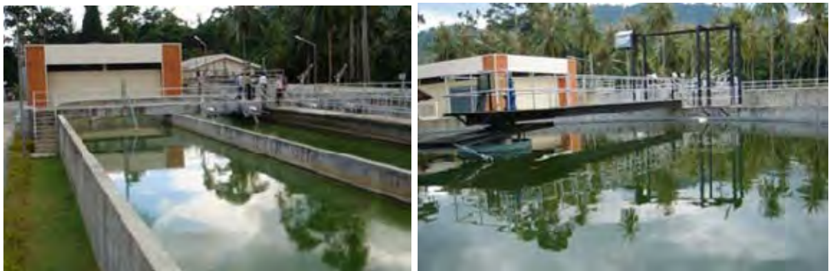
FIGURE 13-23 : Lamai - Hau Thanon Wastewater treatment plant
