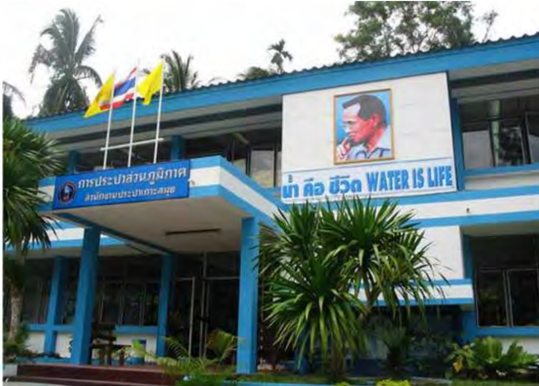
FIGURE 9-28 : Provincial Waterworks Authority of SAMUI Island.
