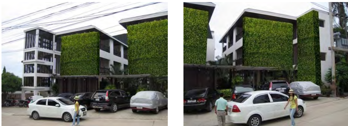
FIGURE 5-36: Private buildings after improvement by using Bio-façade
