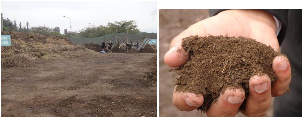
Figure 15: Composting plant run by the Army
