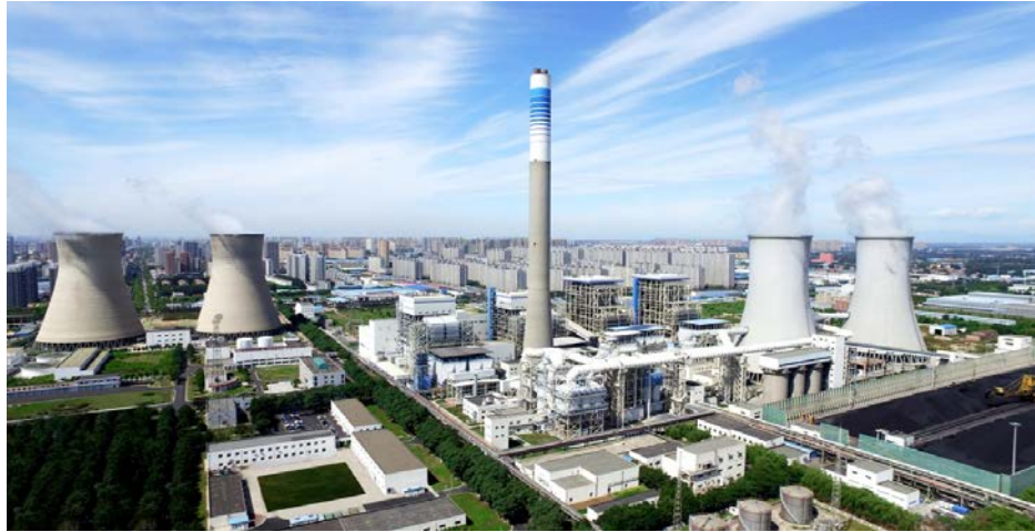
Figure 7-5 Panorama of Hebei Sanhe Power Plant
