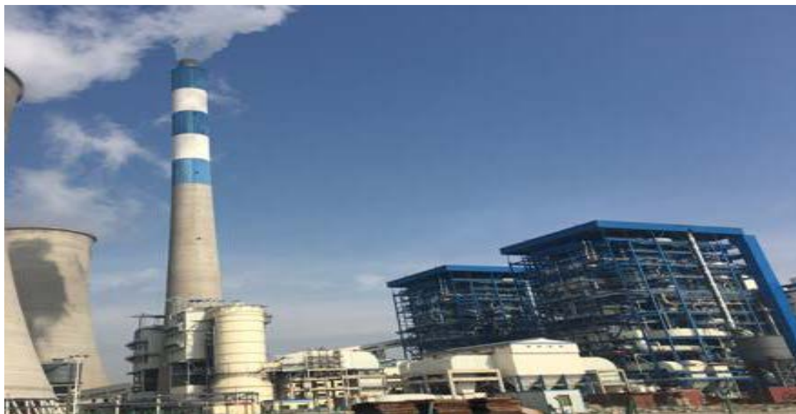
Fig. 5-6 Xuzhou Mining of Hua Mei Thermo-Electric Power
