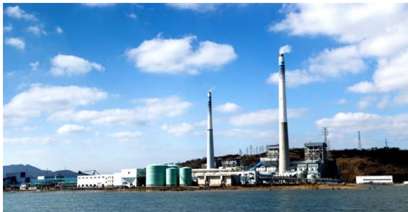
Figure 7-3 Panorama of Zhejiang Zhoushan Power Plant
