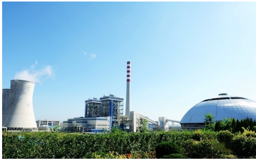
Figure 6-9 A Bird View of Dalian Development Zone Power Plant
