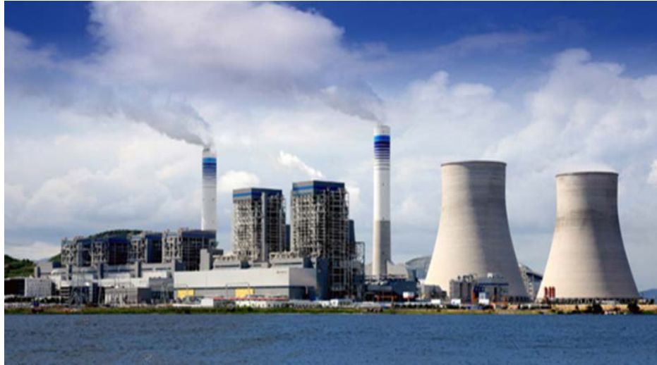
Figure 4-9 A Bird View of Ninghai Power Plant
