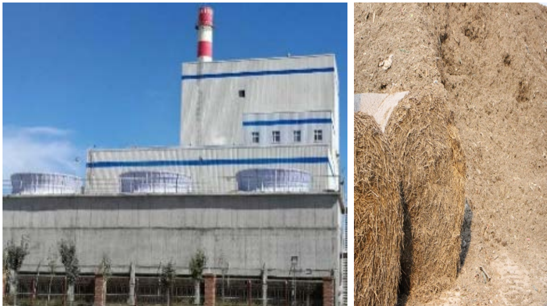
Fig. 5-9 30 MW CFB Boiler with Pure-fired Corn Straw (Qian'an Biopower Plant in Jilin Province)
