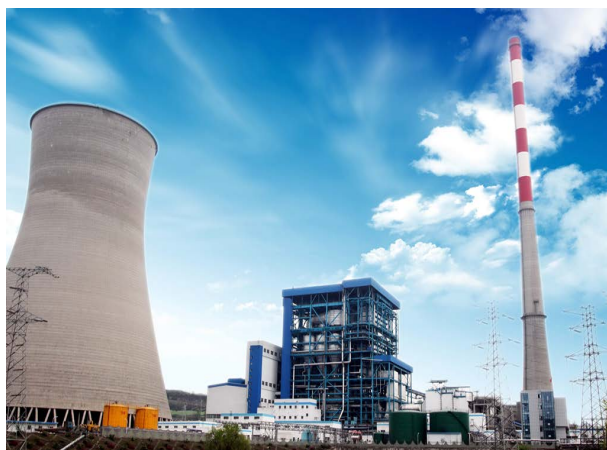
Fig 5-4 Baima 600MW CFB boiler
