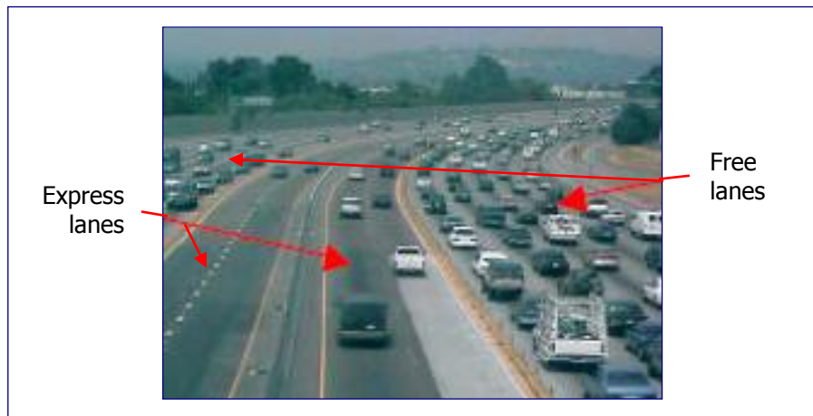
Figure 18. Express and general purpose lanes of SR 91
