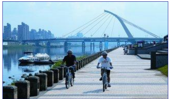
Figure 36. Riverside bicycle lane in Taipei. (Photo: Taipei City Government)
