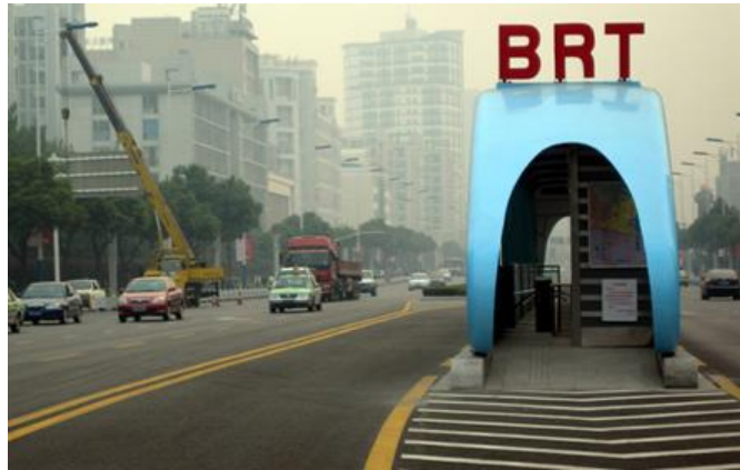
Figure 32. BRT Station in Changzhou. (Photo: www.chinabrt.org )
