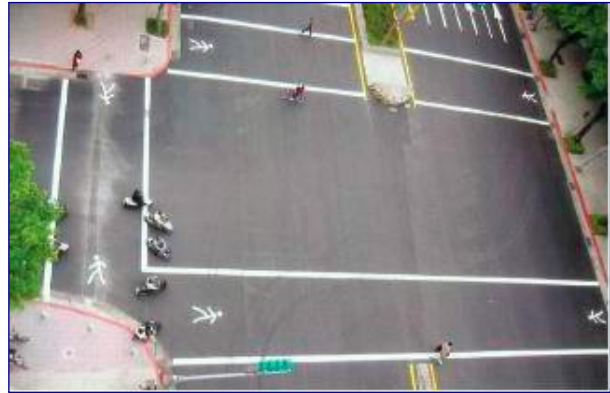
Figure 22. Parallel line pedestrian crossings in Taipei City.
