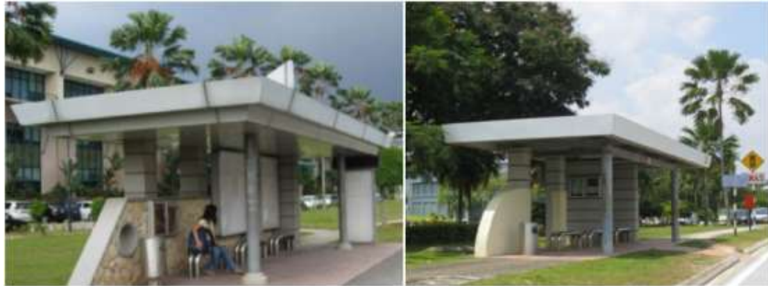
Bus shelters with solar photovoltaic (Cyberview Sdn. Bhd.)
