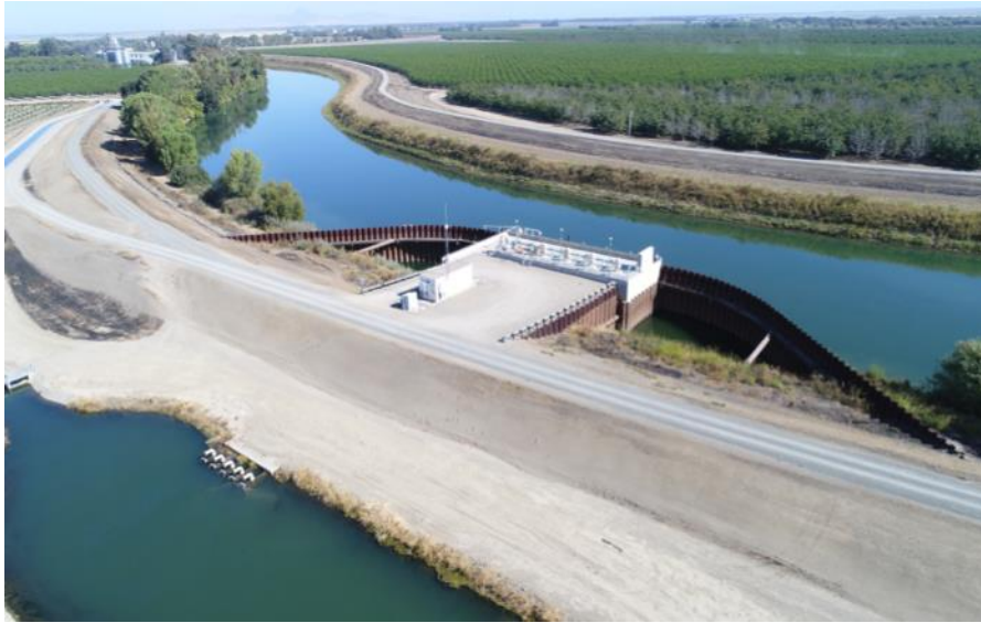
Figure 9. Poundstone Pumping Plant.
