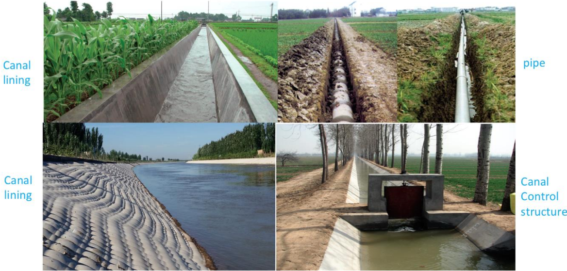
Figure 18. Engineering works to save water during conduction and control.
