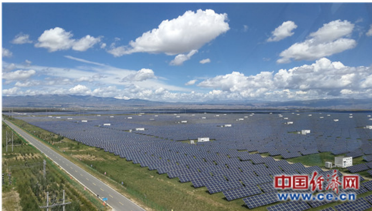
Fig. 3-2.3 PV Power Station in Gonghe County, Hainan State, Qinghai Province, China
