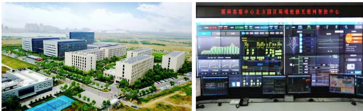
Fig. 3-5.1 Smart Integrated Energy Microgrid in CSC
