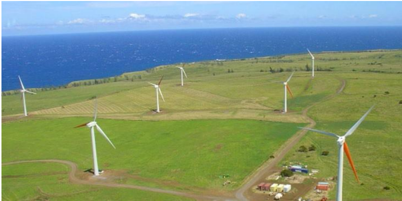
Figure 38 - Hawi Renewable Wind Farm [178]
