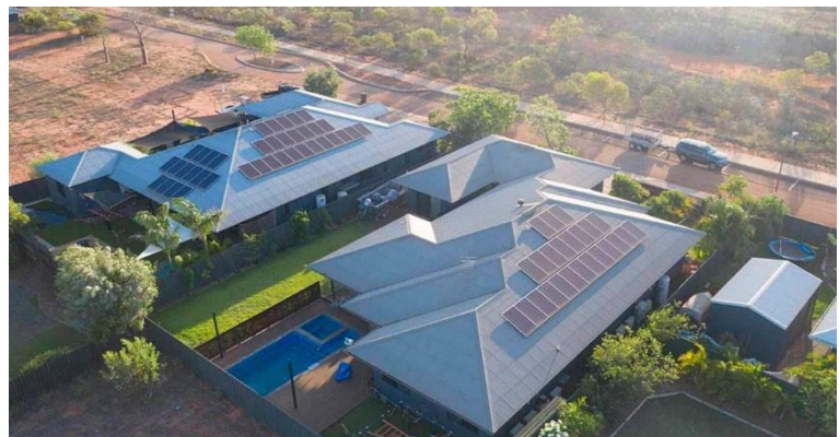
Figure 3 - Distributed Residential Solar - Onslow, Western Australia [160]
