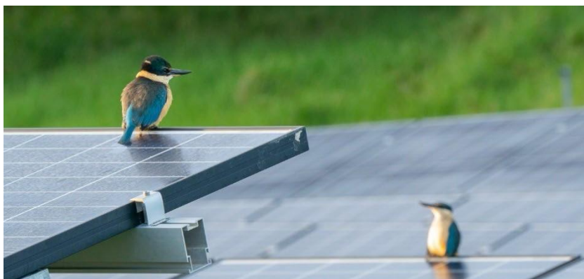
Figure 26 - Native birds on the solar arrays [170]
