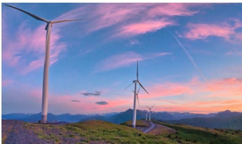
Figure 33 - Kodiak Island Pillar Mountain wind turbines (9 MW) [1]
