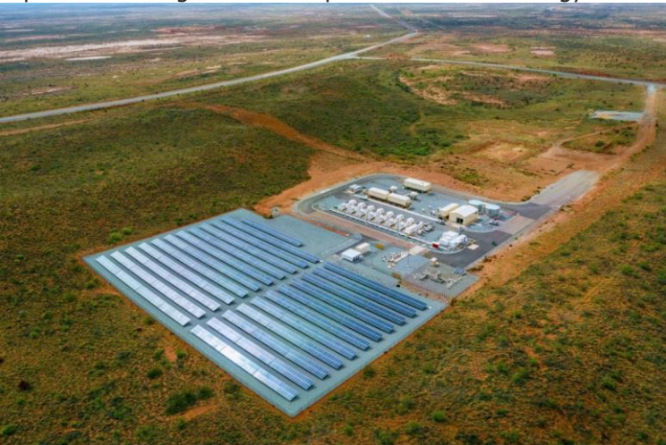
Figure 20 - Onslow Solar Farm [166]
