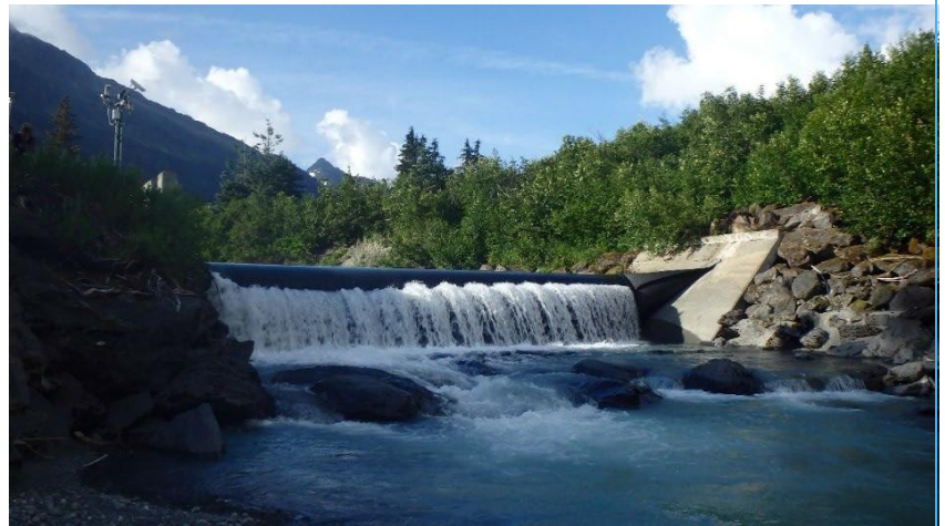
Figure 35 - Power Creek Hydro Facility [159]
