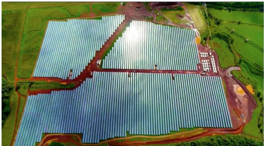
Figure 30 - Tesla 13 MW solar farm and storage on Kaua'i island [173]
