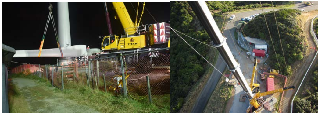
Figure 6: The new Brooklyn Turbine under construction in 2016. Note the predator proof fence in the left of the left hand photo and on the right of the right hand photo. The Brooklyn Turbine is right next to the most significant bird sanctuary in New Zealand.
