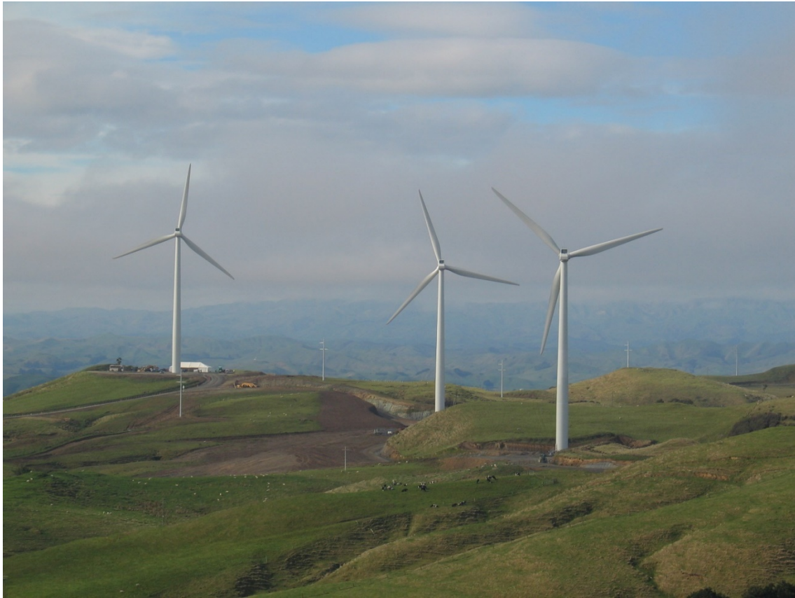
Figure 11: Te Apiti Windfarm.
