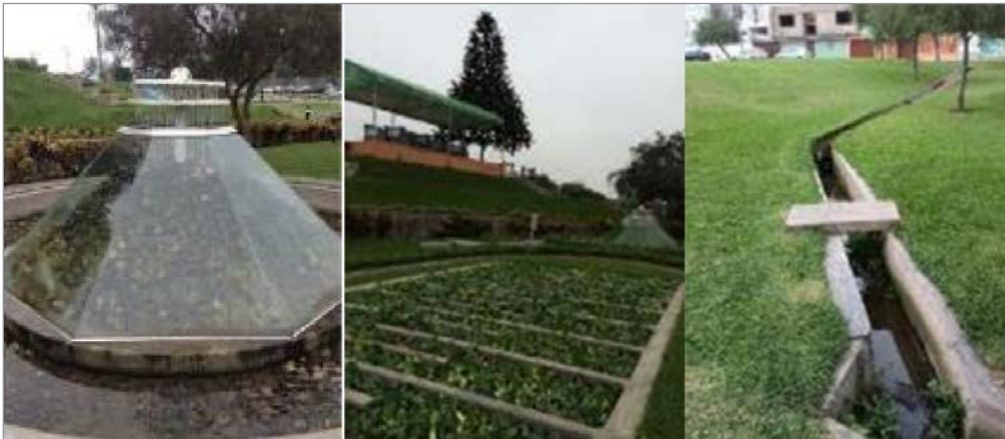
Figure 8-4: Biofiltration Water Treatment System on Irrigation Calans in San Borja
