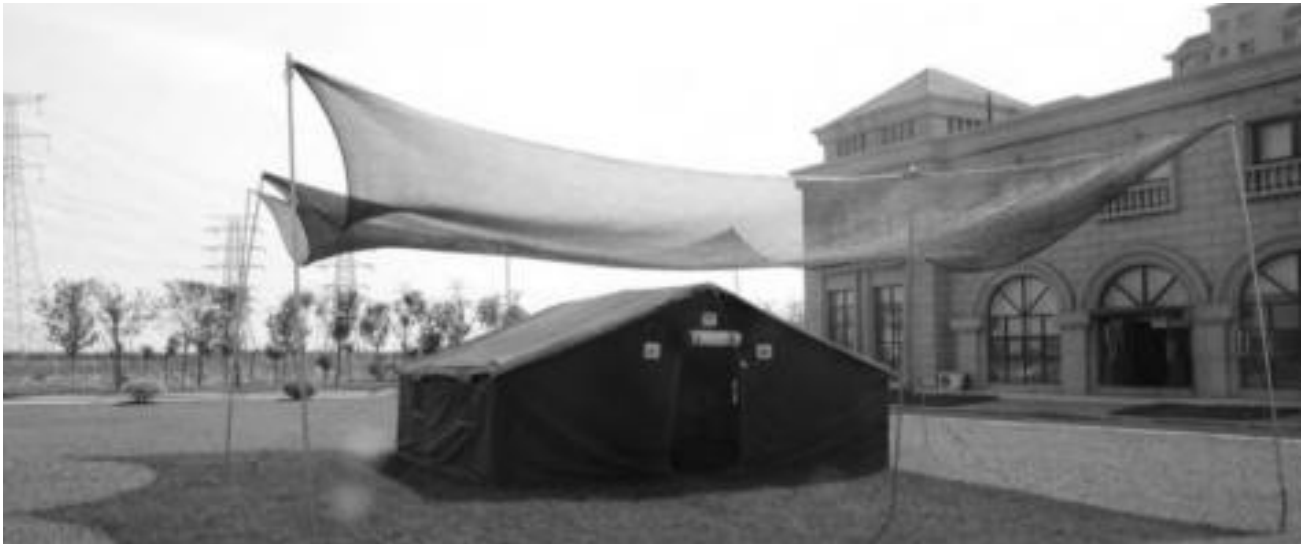
Fig. 2.6 Shade net setting method
