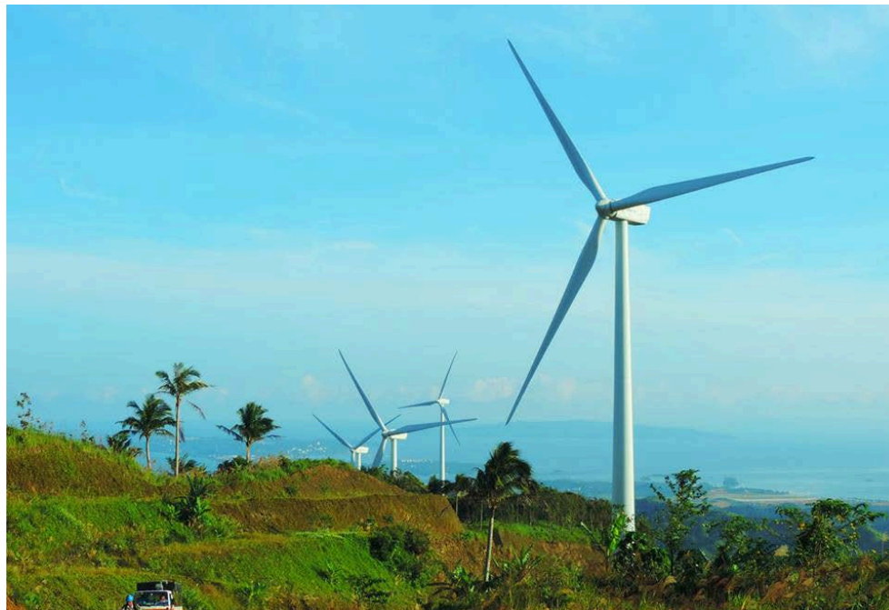
Turbines in the Nabas Wind Farm
