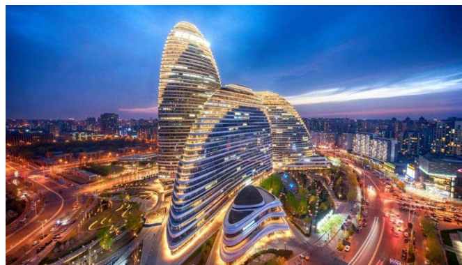
Figure 135: Wangjing Soho towers, Beijing
