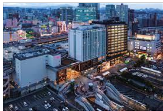
Figure 3: Sendai Station in Sendai, Japan. Source: JICA
