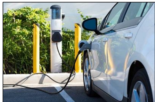
Figure 11: A BEV charges at a new charging station in Sydney, AU.
