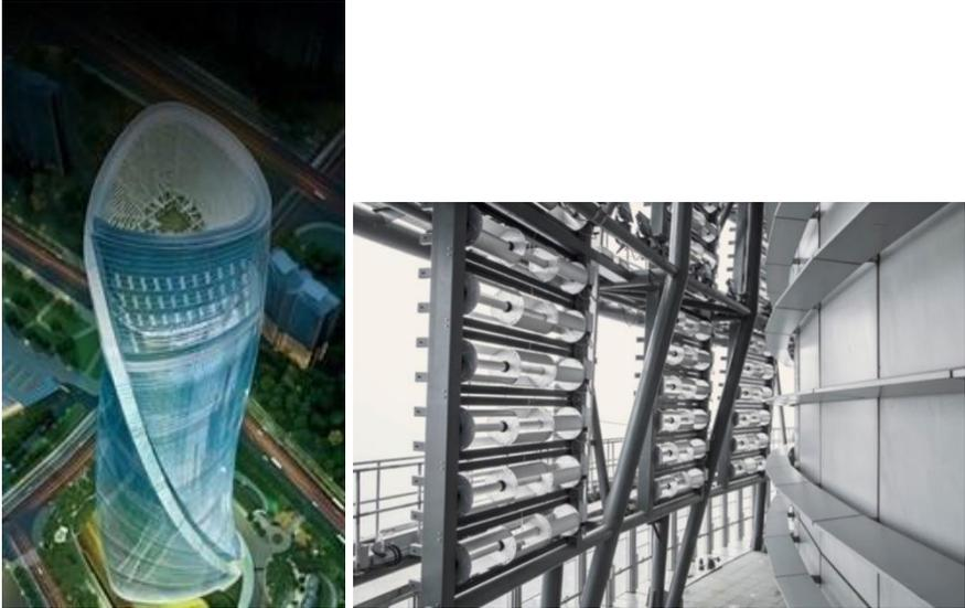
*Figure 92: Shanghai Tower (left) and its installed wind turbines (right)*
