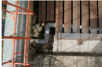
Fig. 2.1-26. Methane gas pipe (LEFT) and Gas range using methane gas (RIGHT) Source: NSRI
