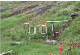
Methane Gas Distribution Piping
