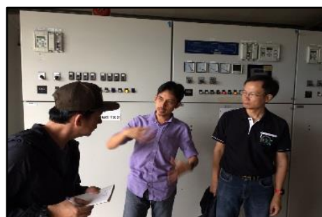
Figure 20 Visiting the Solar PV at SunEdison
