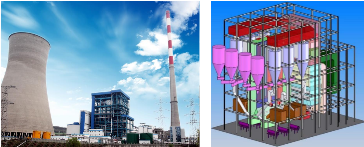
Figure 2- 2 Baima 600MW circulating fluidized bed boiler
