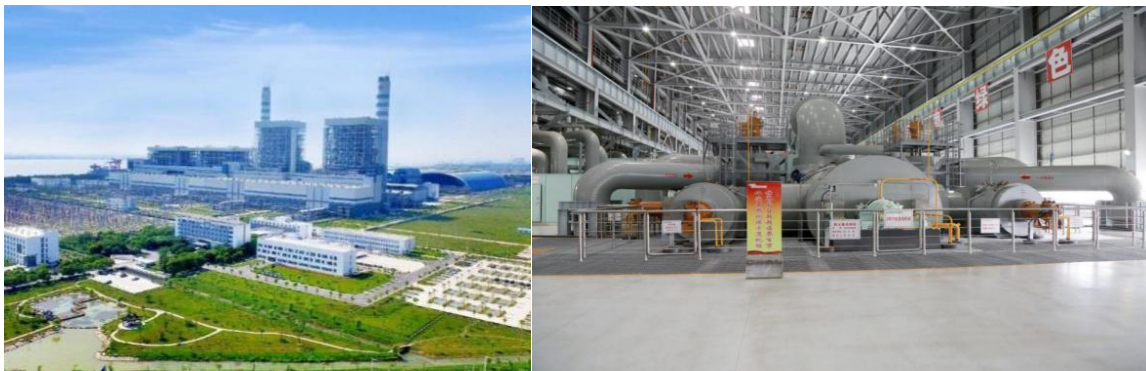
Figure 2- 1 Taizhou Power Plant and the second-stage secondary reheat turbine
