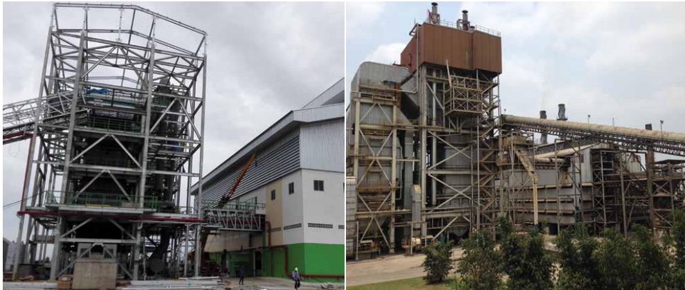
Figure 2- 14 Coconut Power Plant, Thailand Figure 2- 15 Veracruz Sugar Power Plant, Mexico
