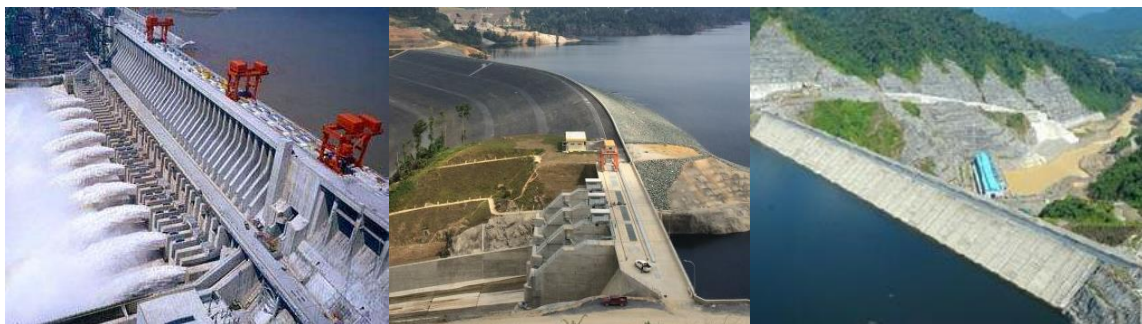
Figure 2- 10 Three Gorges Hydropower Station Figure 2- 11 Hulu Hydropower Figure 2- 12 Semangka Hydropower Station
