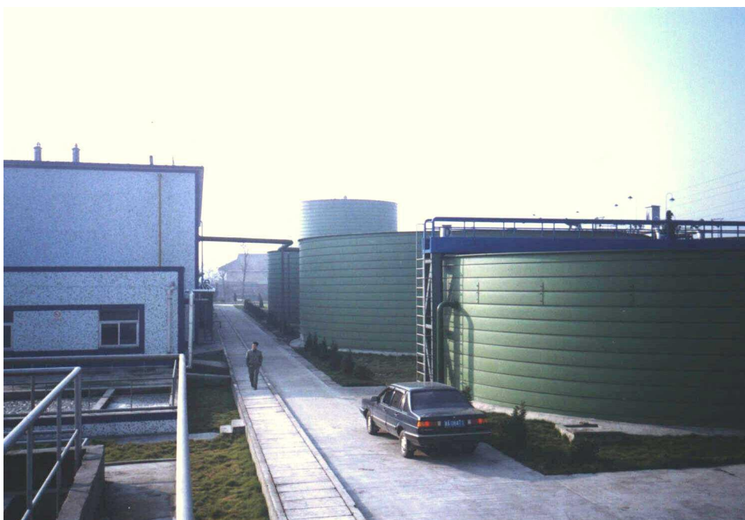
Biogas system for treating wastewater on the 200,000-pig Hangzhou Dengta Farm. Photo courtesy of Hangzhou Energy & Environment.
