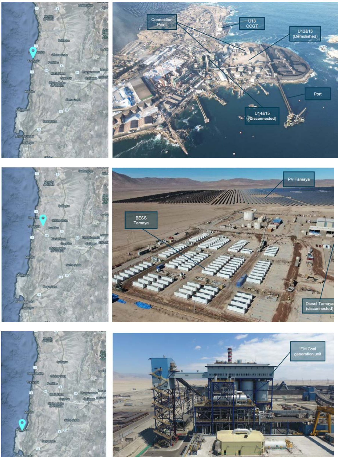
Figure 1 Location of thermal complexes Tocopilla, Tamaya and Mejillones
