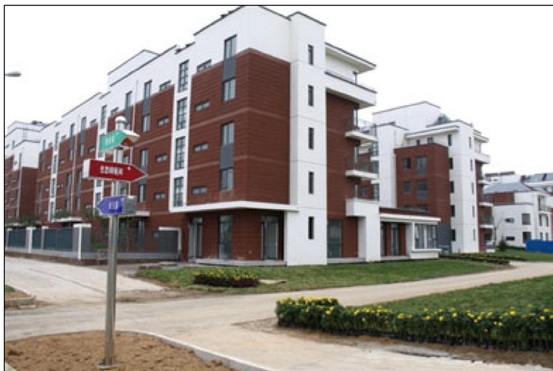
Figure 20. First green housing project in Caofeidian Eco-city
