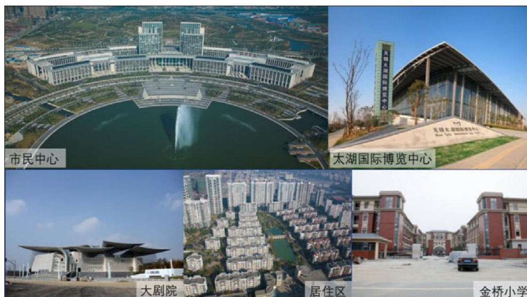
Figure 22. Construction of Taihu New Town
