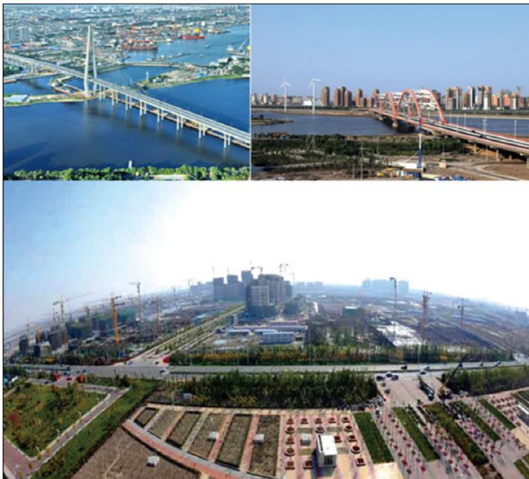
Figure 17. Construction of Sino-Singapore Tianjin Eco-city
