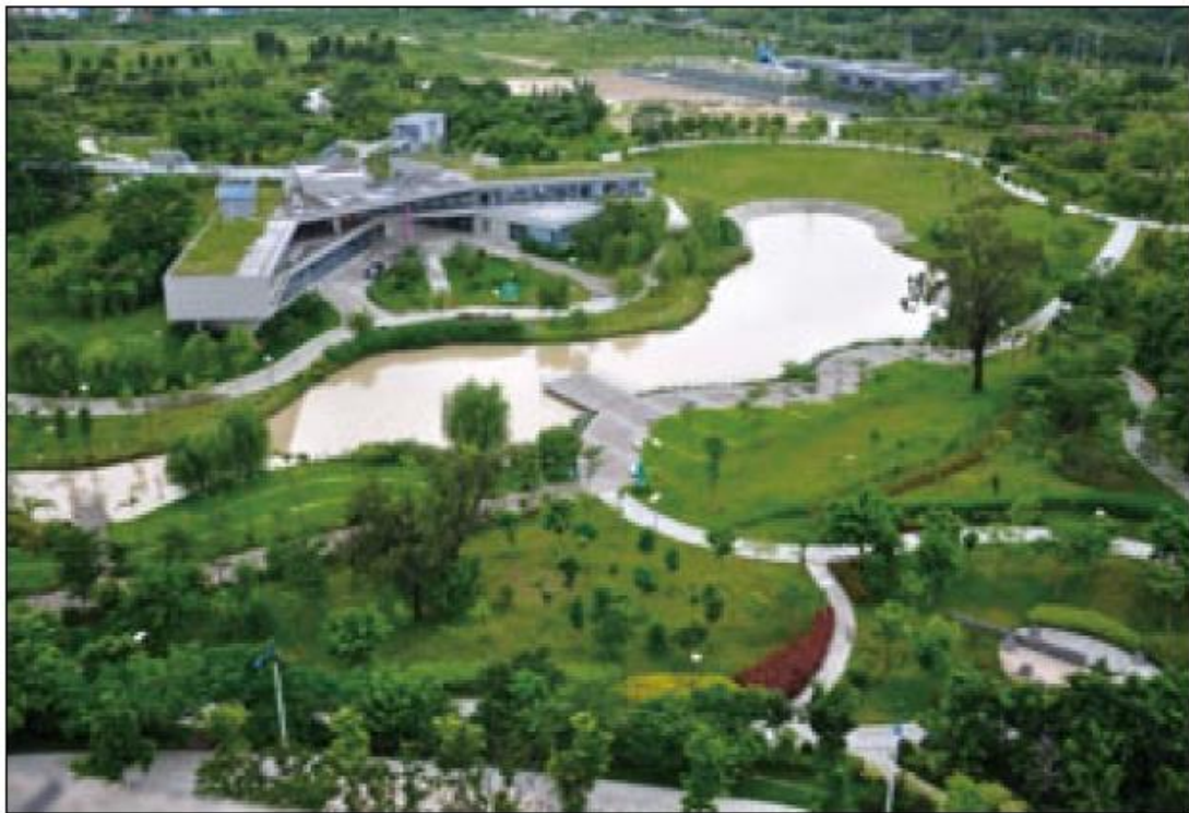
Figure 24. Low impact treatment of river basins and green building construction in Pingshan New District
