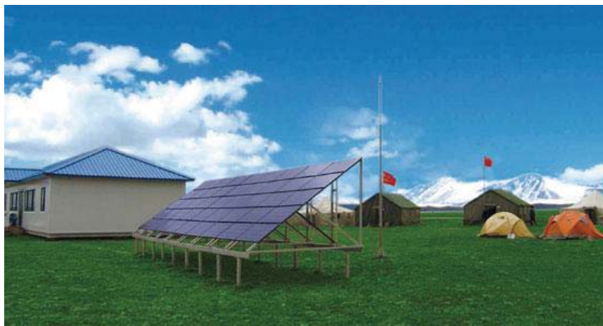
Fig. 2-23 Photovoltaic off-grid system
