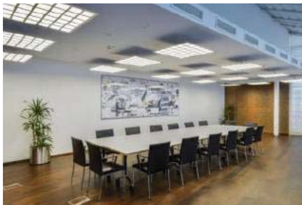
Fig. 4-9 Energy-saving lighting system
