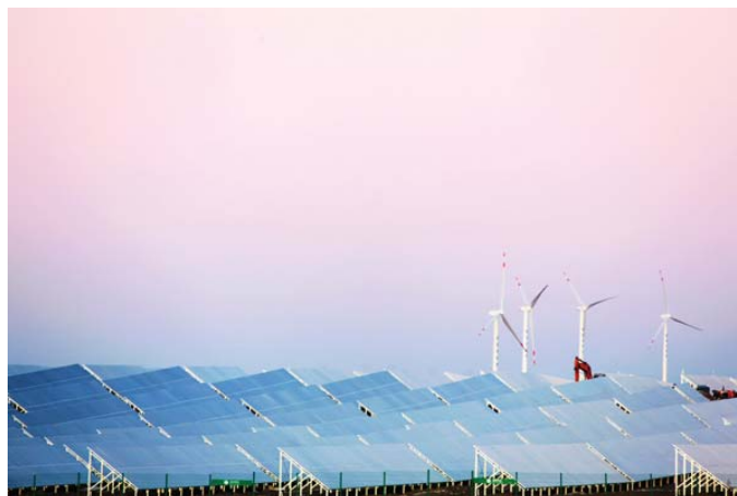
Fig. 3-12 China National Wind-solar Energy Storage Demonstration Project
