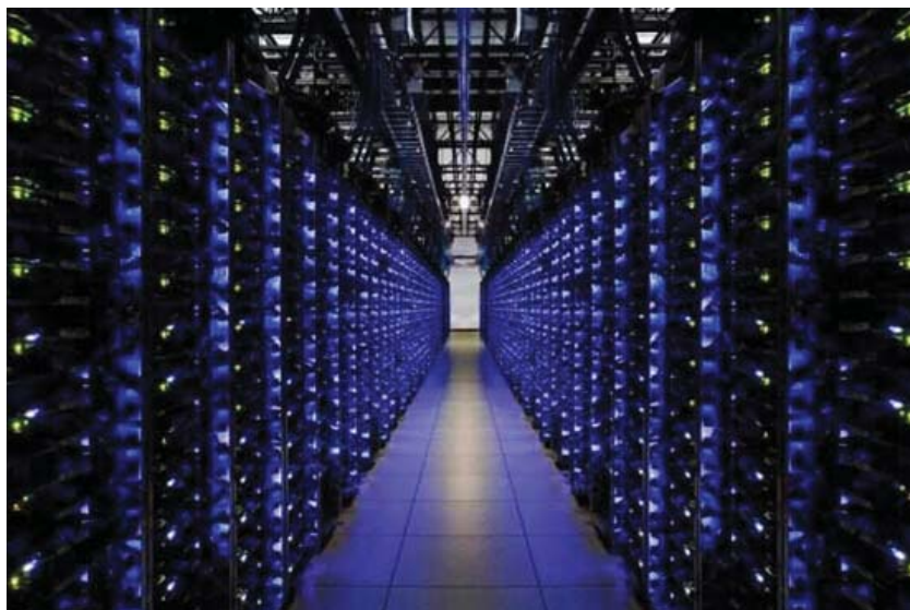
Fig. 5-8 Distributed energy efficiency management micro grid of Google Data Center
