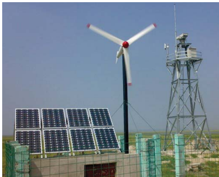
Fig. 2-15 Wind-solar hybrid system
