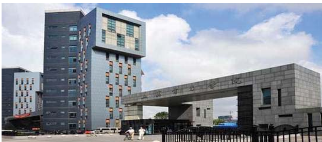
Fig. 3-3 Demonstration and research center of smart micro-grid in Shanghai
