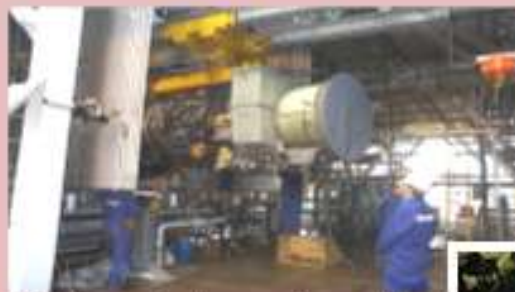
Replace the motor LM6000
