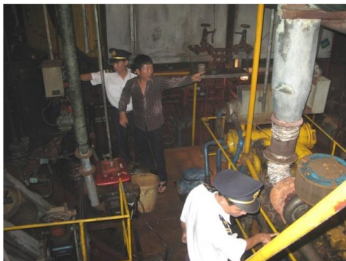
Figure 2-95: International ship being inspected before leaving port
