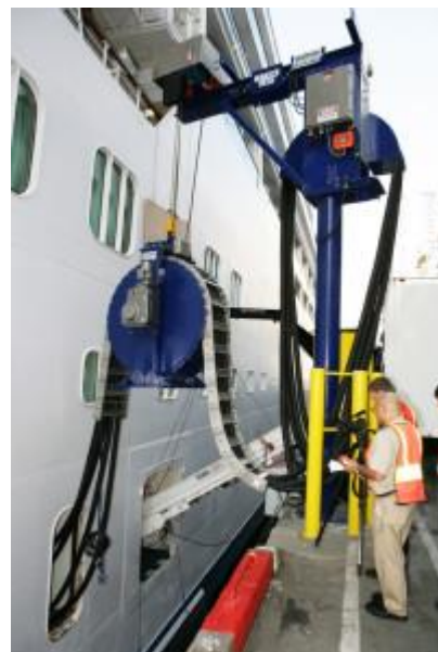
Figure 2-14: Pulling the power cable into the ship
