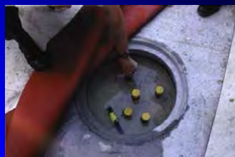
Surface top part of the borehole and double u-tubes. They will be connected to a heat-pump.
