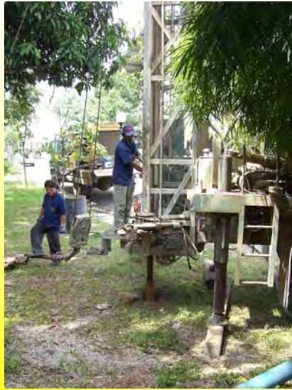
Drilling of heat exchange borehole, 2006.10.17
