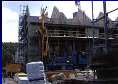
Construction of an apartment complex and a drilling machine for borehole heat exchanger
