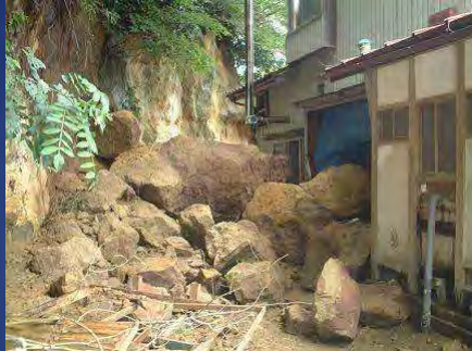
Slope failure caused by earthquake. July 2003 Miyagi
