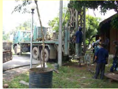
Drilling of heat exchange borehole, 2006.10.17
