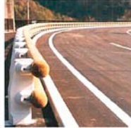
The Wooden Guardrail
