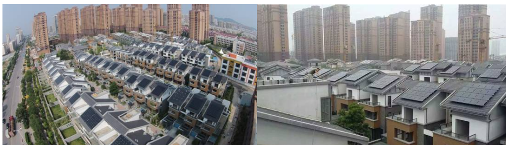
Fig. 5-4 Shoufu Villa BAPV Project
