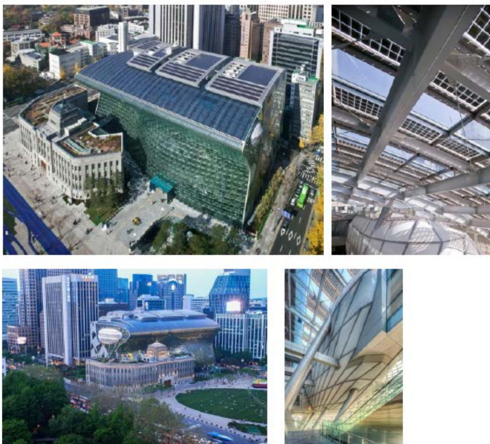
Fig. 5-10 Seoul City-Hall rooftop and curtain wall BIPV
