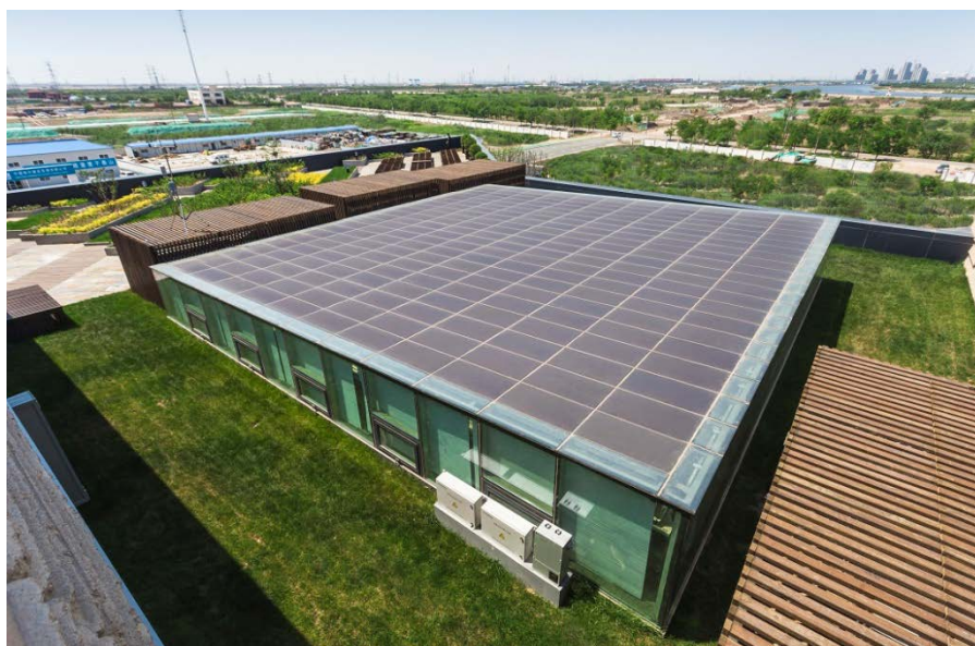
Fig. 2-9 Industrial building with BMPV
