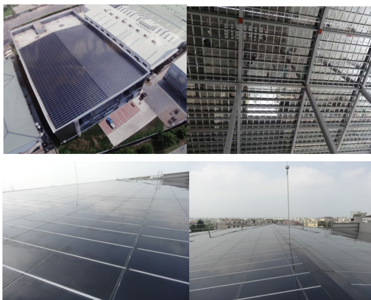
Fig. 5-9 Jinhuaqing factory buildings roofing BIPV project in Chinese Taipei
