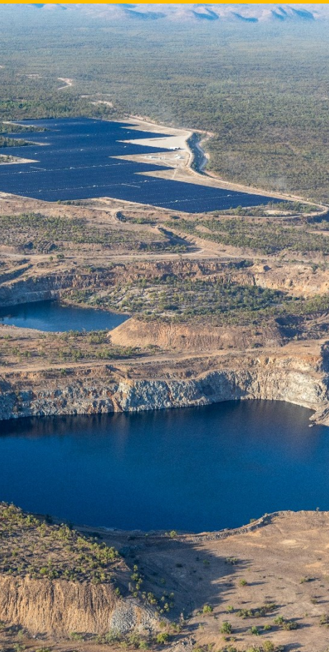
Kidston Solar Farm and PSH System, North Queensland (Source: Genex Power)
