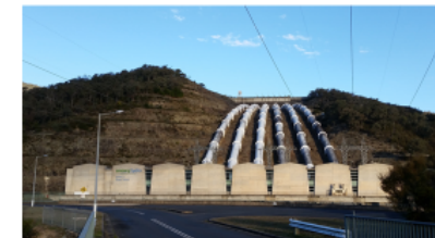
Tumut 3 pumped storage power station, 1,500 MW capacity, Australia © J Pittock
