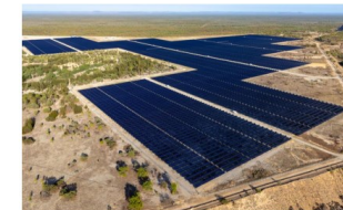
Kidston 50MW Solar Project
