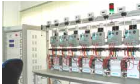
Electronic test bench with Common Mode Rejector unit to enable testing of three phase meters even with voltage link closed
