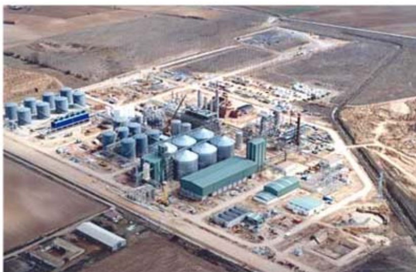
Figure 3.15 Site View of Abengoa's BCyL Biomass Plant
