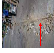
Cabling from control room to fuel dispenser
