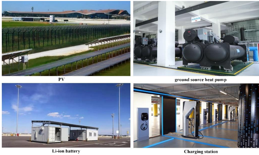
Fig. 3-19 DERs and charging station in Daxing Airport
