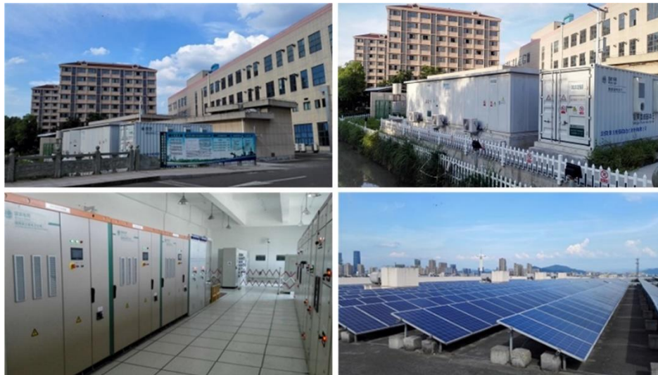
Fig. 3-16 Part of the Shangyu hybrid AC/DC MG project
