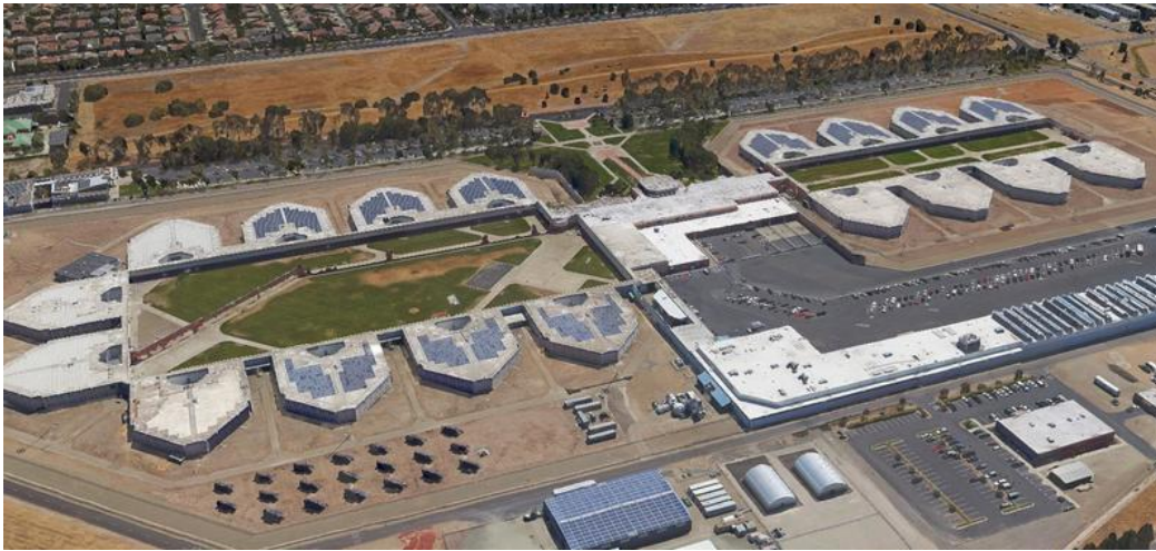
Fig. 3-1 Top view of Santa Rita Jail
